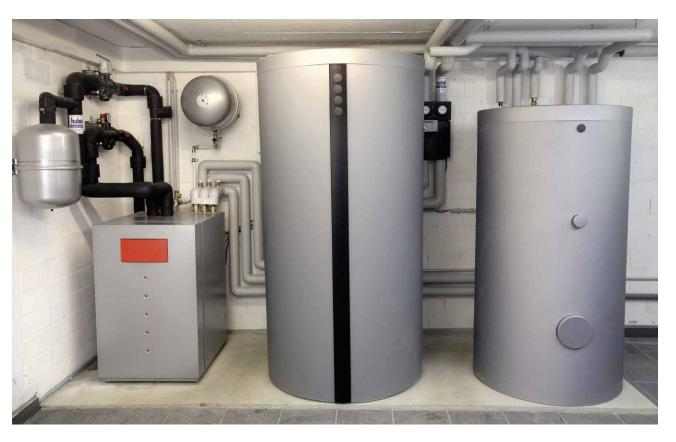
Figure 127: Heat pump with potable hot water storage tank
