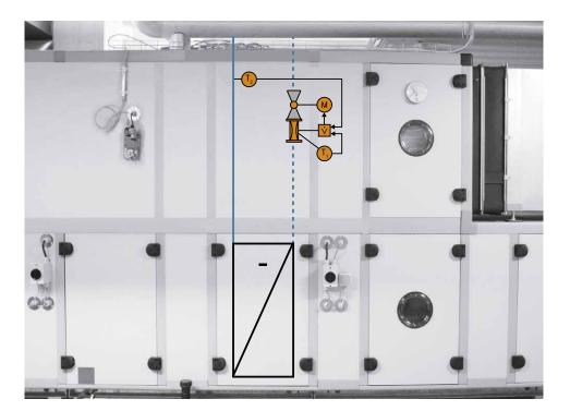
Figure 57: Example of a typical Air Handling Unit (AHU) Cooling Coil with EV
