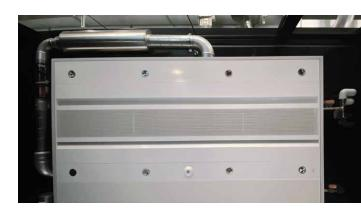
Figure 91: Ceiling integrated chilled beam with air and chilled water supply
