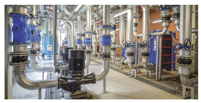
Figure 68: Picture of a Heat Exchange Station
