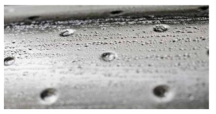
**Figure 95:** Condensation of humid air on the cold coil surface. The supplied cooling water needs to be above indoor dew point to prevent condensation
