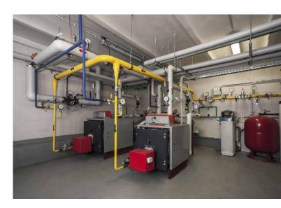
Figure 126: Condensing gas boiler
