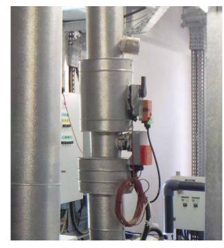
Figure 90: The supply of the Fancoil Units is equipped with the Belimo Energy Valve $^{\text{\tiny M}}$
